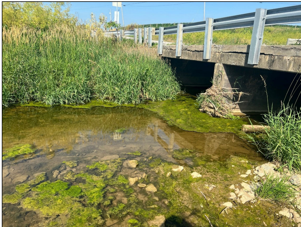
Upstream face of culvert
