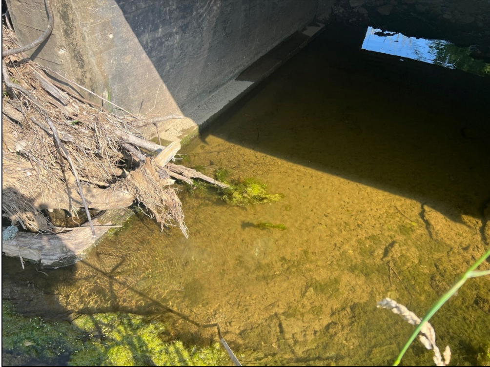
Footing on bedrock
