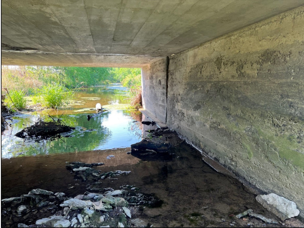
Looking upstream through middle barrel
