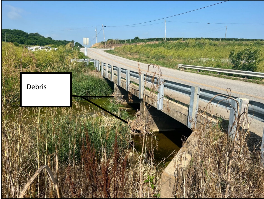
Upstream face of culvert
