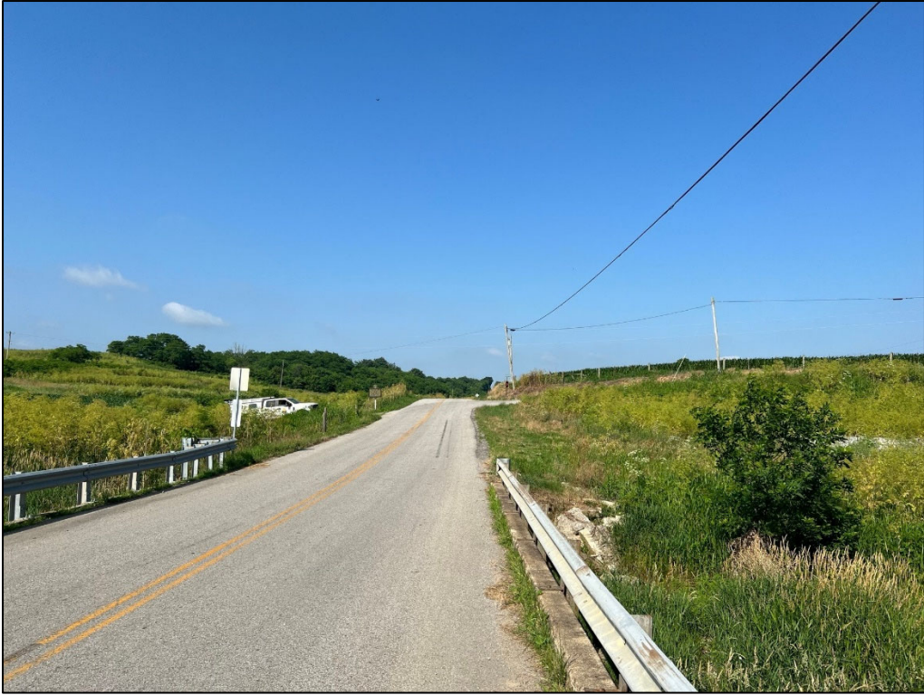
Looking south from culvert
