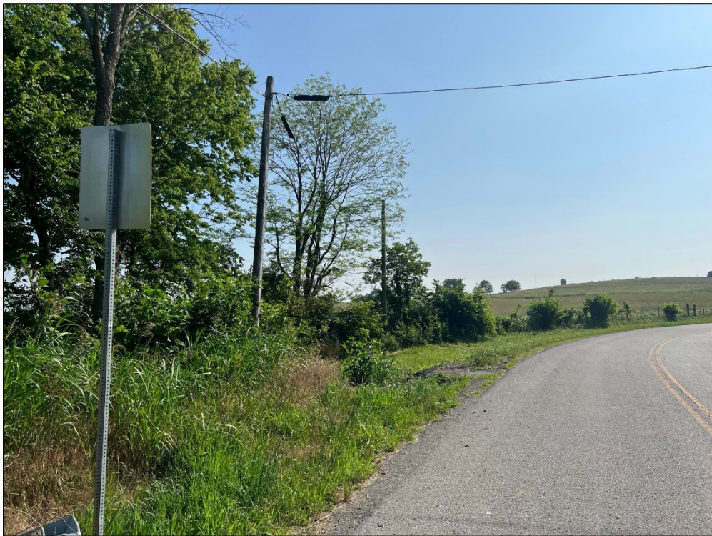
Utility poles about 40' north of culvert
