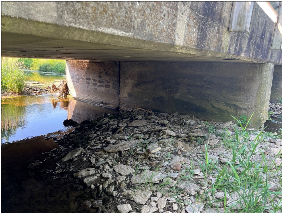
Downstream face of culvert
